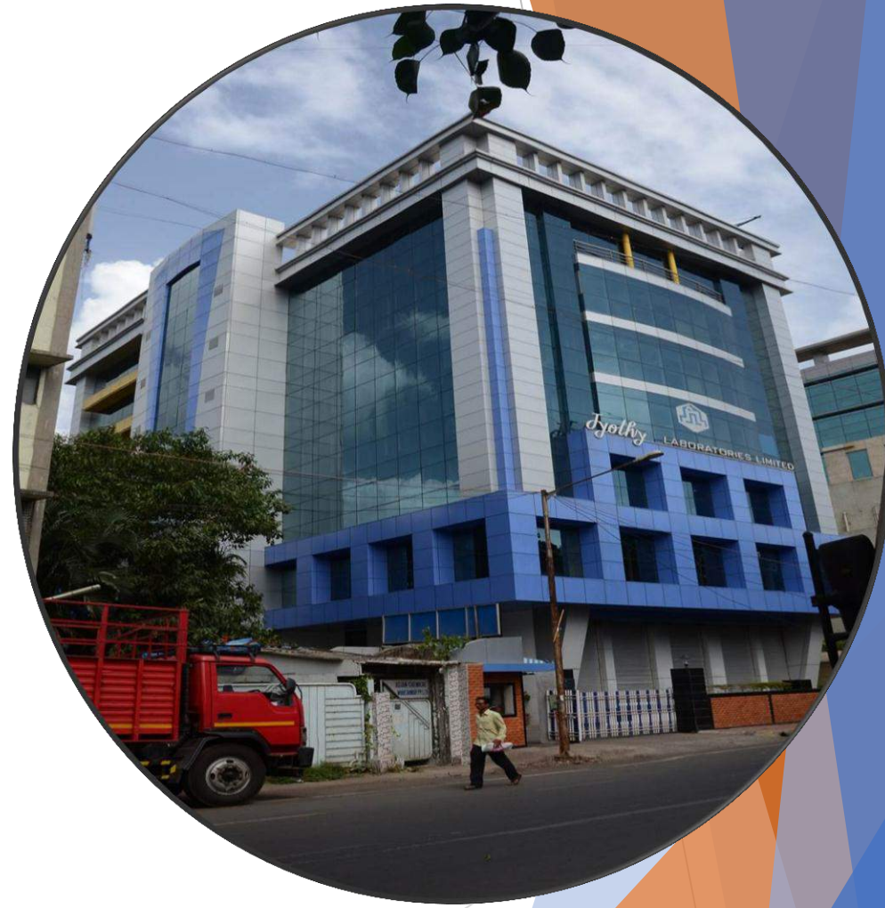
Office Building for Arena Enterprises at Kondivita, Andheri East, Mumbai
